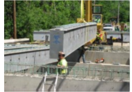
The hybrid-composite beam uses a tested technology to make structures lightweight, strong, and corrosion resistant.
